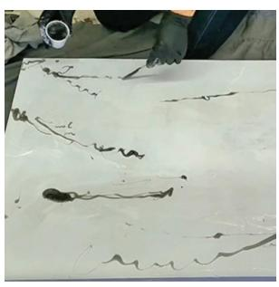
Drizzle lines of light gray epoxy in random locations on the top and down the sides of the white epoxy surface. It's best to keep the lines going in a similar direction to mimic marble's natural lines. Use a clean tongue depressor to control the line of light gray epoxy as you apply it.
