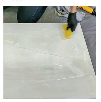
Pour the white mixed epoxy across the surface in an 'S' shape. Use a clean plastic spreader to distribute the epoxy until it covers the top and surfaces at a uniform depth of about 1/8".
