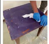
Clean the table top by wiping with a rag wetted with \*\*acetone or denatured alcohol\*\*.
