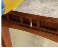
Remove the tape. Sand any rough edges with 120 grit, and wipe with acetone.
