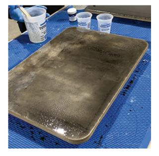
Pour a thin 1/16" seal coat of black mixed epoxy onto the surface. Use a spreader to spread the epoxy evenly. WAIT FOR THE EPOXY SEAL COAT TO SET UP AND BE TACK-FREE BEFORE APPLYING YOUR FLOOD COAT. If you wait until the surface hardens completely, sand with 220 grit and remove residue by wiping with acetone, and let dry.
